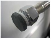
Photo 9. 3/4" Plug in Stainless Steel Flex Hose in Outlet Line
